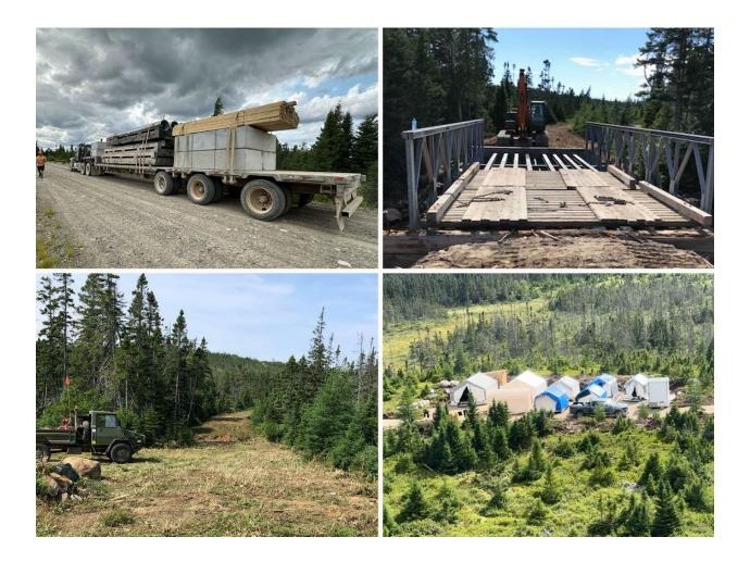
1890 - 1075 West Georgia St. Vancouver, BC, V6E 3C9 info@fanickel.com www.fanickel.com LEADING THE CHARGE TSXV:FAN · OTC:FANCF · FSE:P21 Figure 1: Images showing infrastructure upgrades including road clearing, culverts, and multiple bridge installations giving year-round access to the Project. Bottom right, phase 1 camp established on the Atlantic Nickel Project site.
